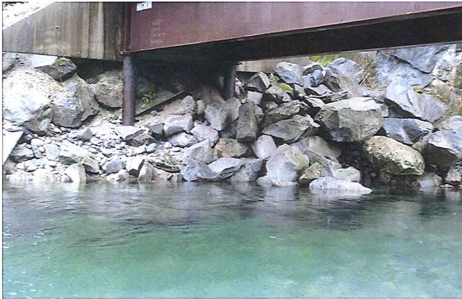
CK2378 Right Abutment
