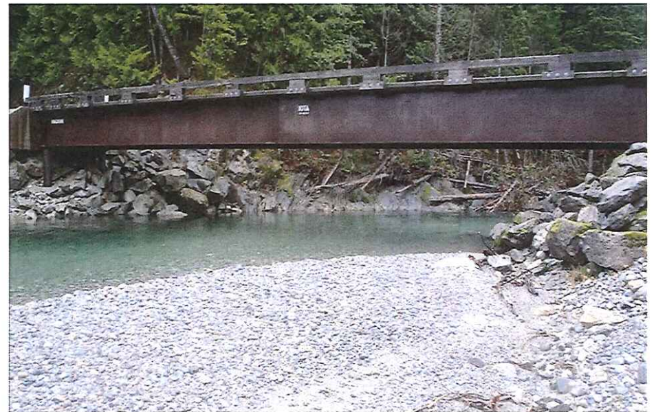
CK2378 From Downstream
