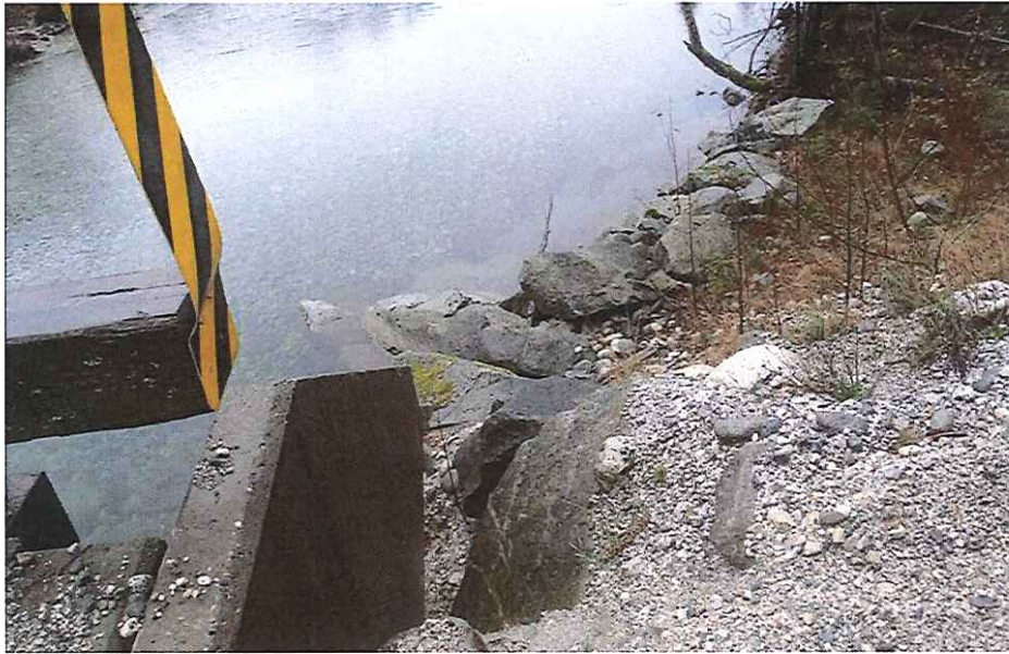
CK2378 Right Abutment fill
