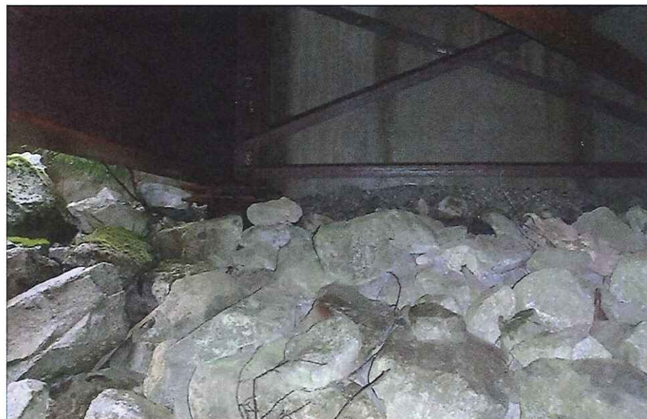
CK2378 Left Abutment
